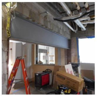
Take a look at the massive steel beam that was installed to provide a new living room space where the old Business Office used to be located.
